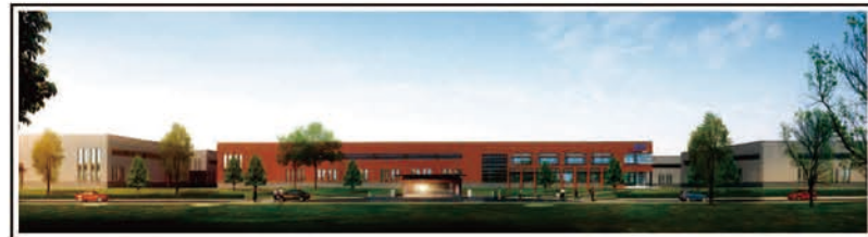
New Facility in Huzhou
